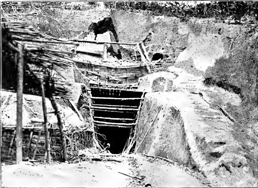
Fig. 3.—OPEN-CUT ON 4-ft. VEIN
